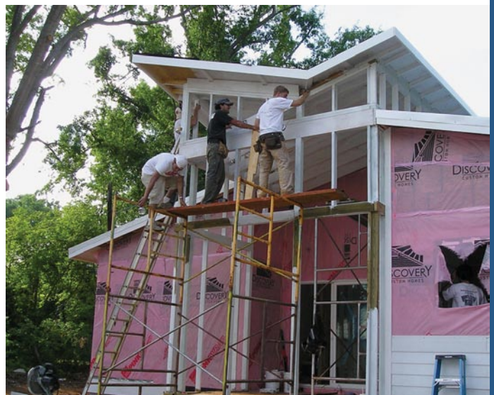
Figure 5. Center bay under construction
