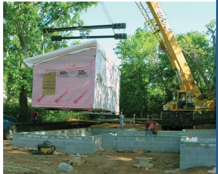
Figure 4. Setting modules on the foundation
