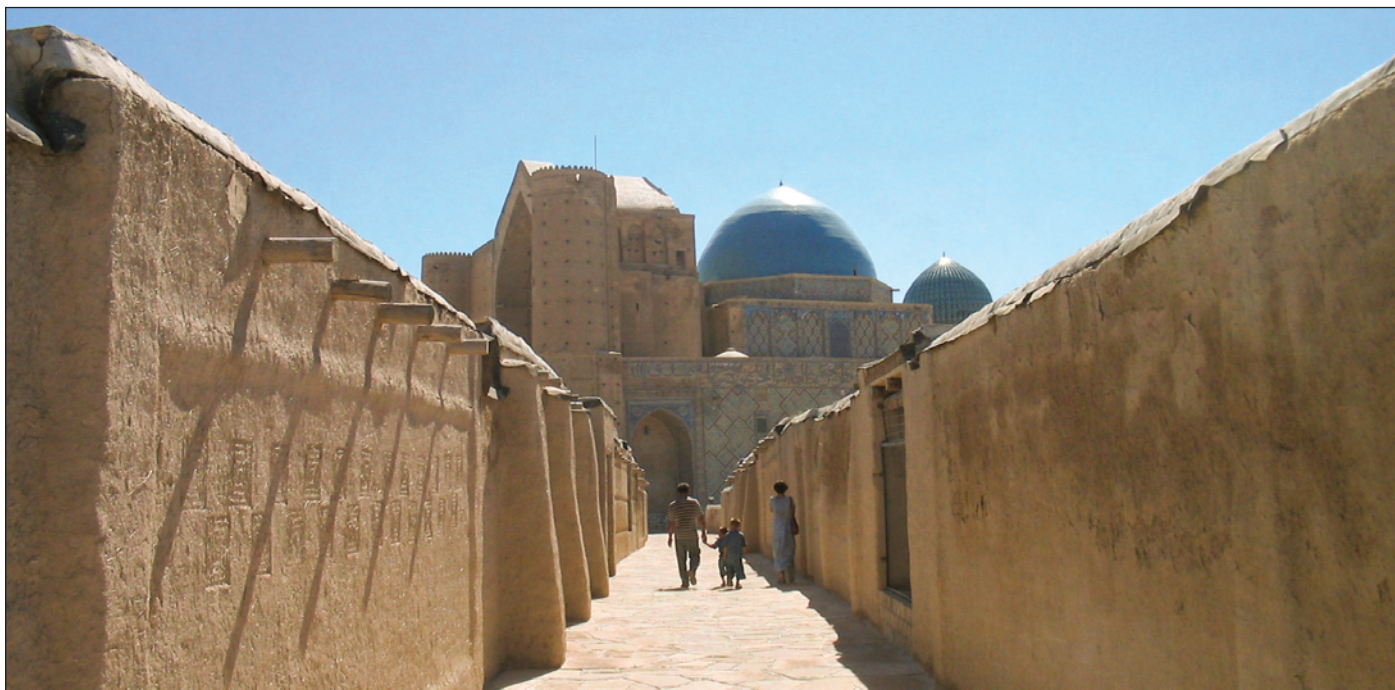
The Shrine of Hojja Ahmet Yasawi in Turkestan City, Kazakhstan, as seen in this June 2004 photo, was begun by the 14 th -century Central Asian ruler Tamerlane to honor this figure in the spread of Islam among Turkish-speaking people. Unfinished, it is visited by hundreds of thousands of Central Asian Muslims each year.
