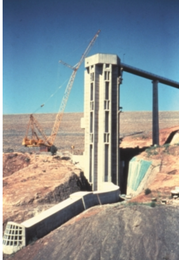
Selective withdrawal intake-tower at Lost Creek Dam, Oregon. Intake ports are each 8 feet wide by 15 feet tall. Distances between ports vary from 55 to 90 feet. Photo taken in 1977 by author.
